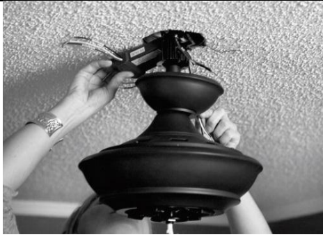
Fig. 2.13: Unscrew the outside nuts of the fan
